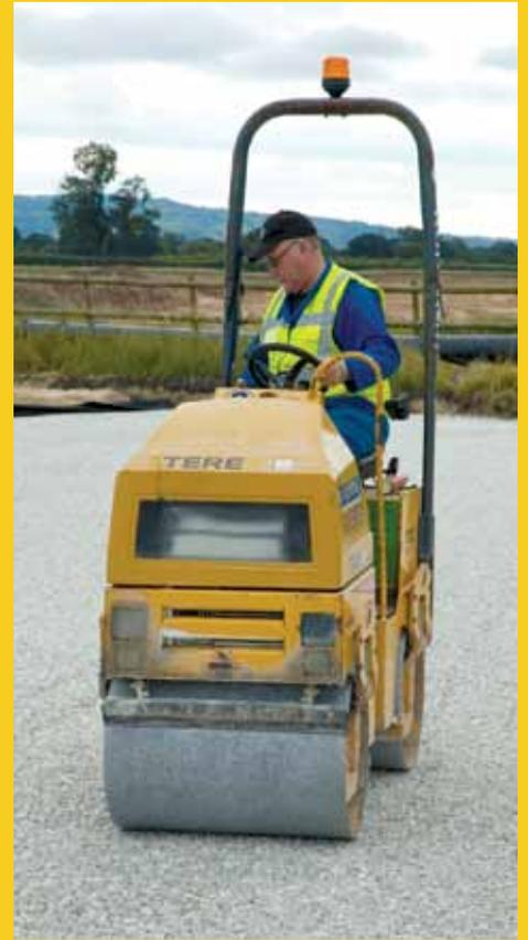
The base layer must be level, with the stones firmly packed together for stability, separated from the riding surface by a suitable porous membrane, and sound enough to withstand heavy impact.
